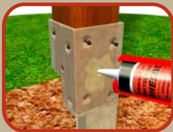
1/2" In With Screws & Glue
